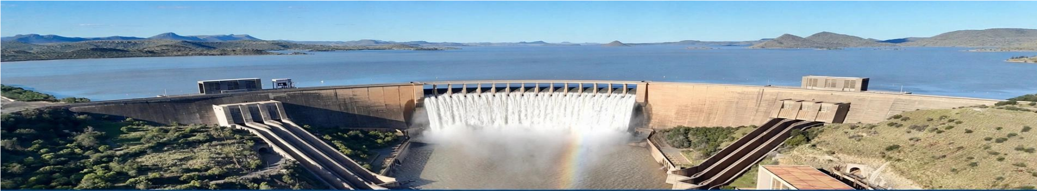
GARIEP DAM • SOUTH AFRICA
